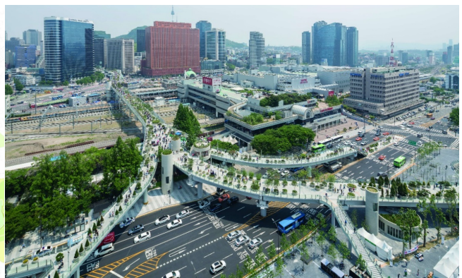
Pic. 5. Seoullo Park Overpass 7071 Skygarden, Seoul (Author Sen Yang) [6]
