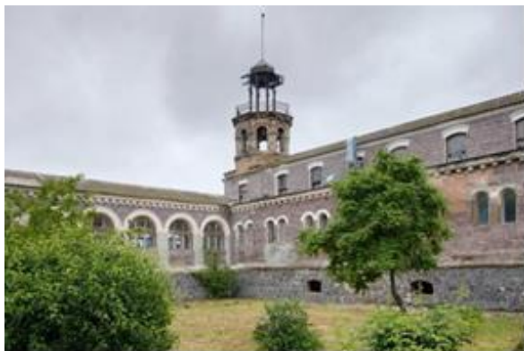
Fig. 8. Inner courtyard of the Kuyalnyk mud bath facility, current condition
