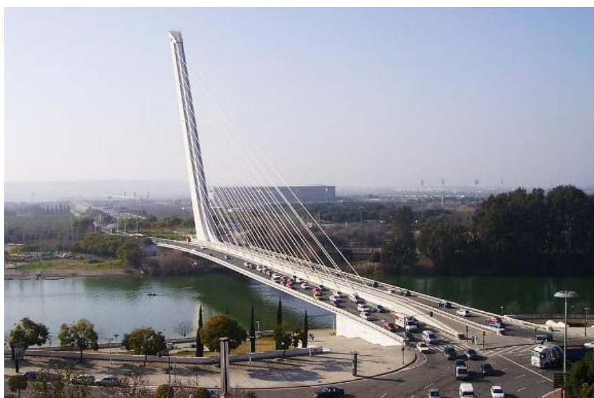
Pic. 2. Al Amilo bridge in Seville, architect Santiago Calatrava, Spain
